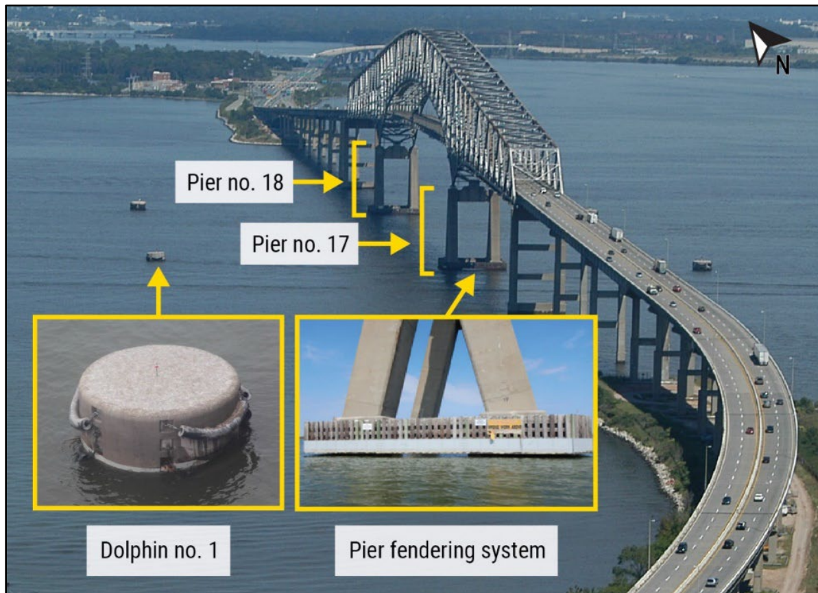
Figure 12. The Key Bridge and the locations of pier nos. 17 and 18. Insets show dolphin no. 1 as well as pier no. 17's fendering-system surrounding. (Background source: MDTA)
